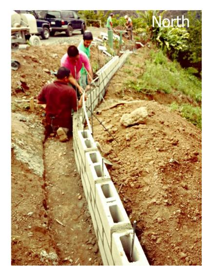
Sixty meters of concrete walls were built, some deeper than others depending on the terrain.
