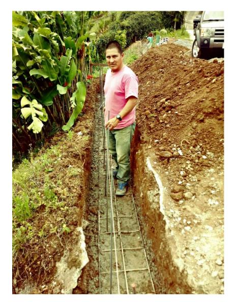
Deep concrete footings were poured over rebar to secure the concrete blocks
