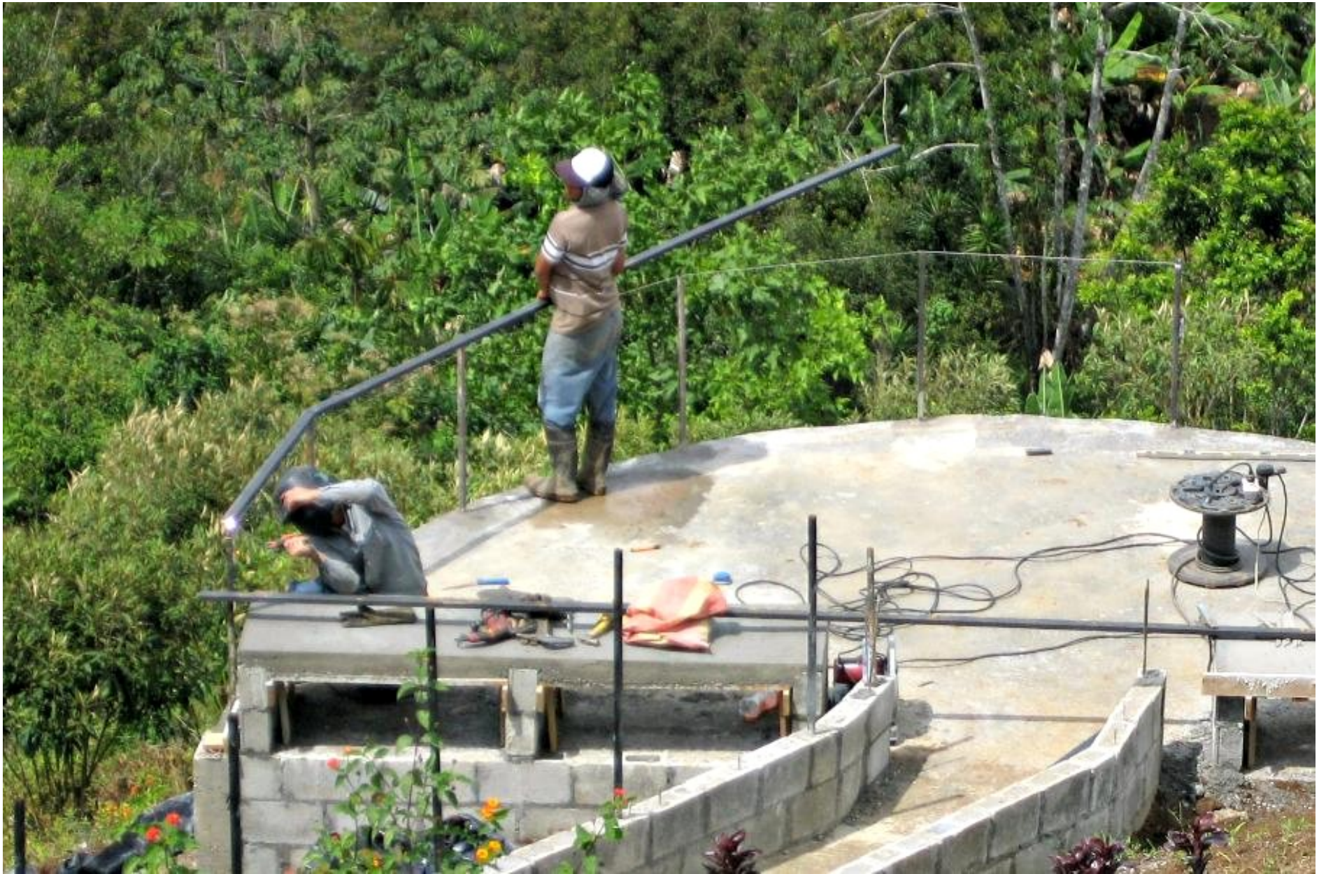
Solderero welding the handrails.
