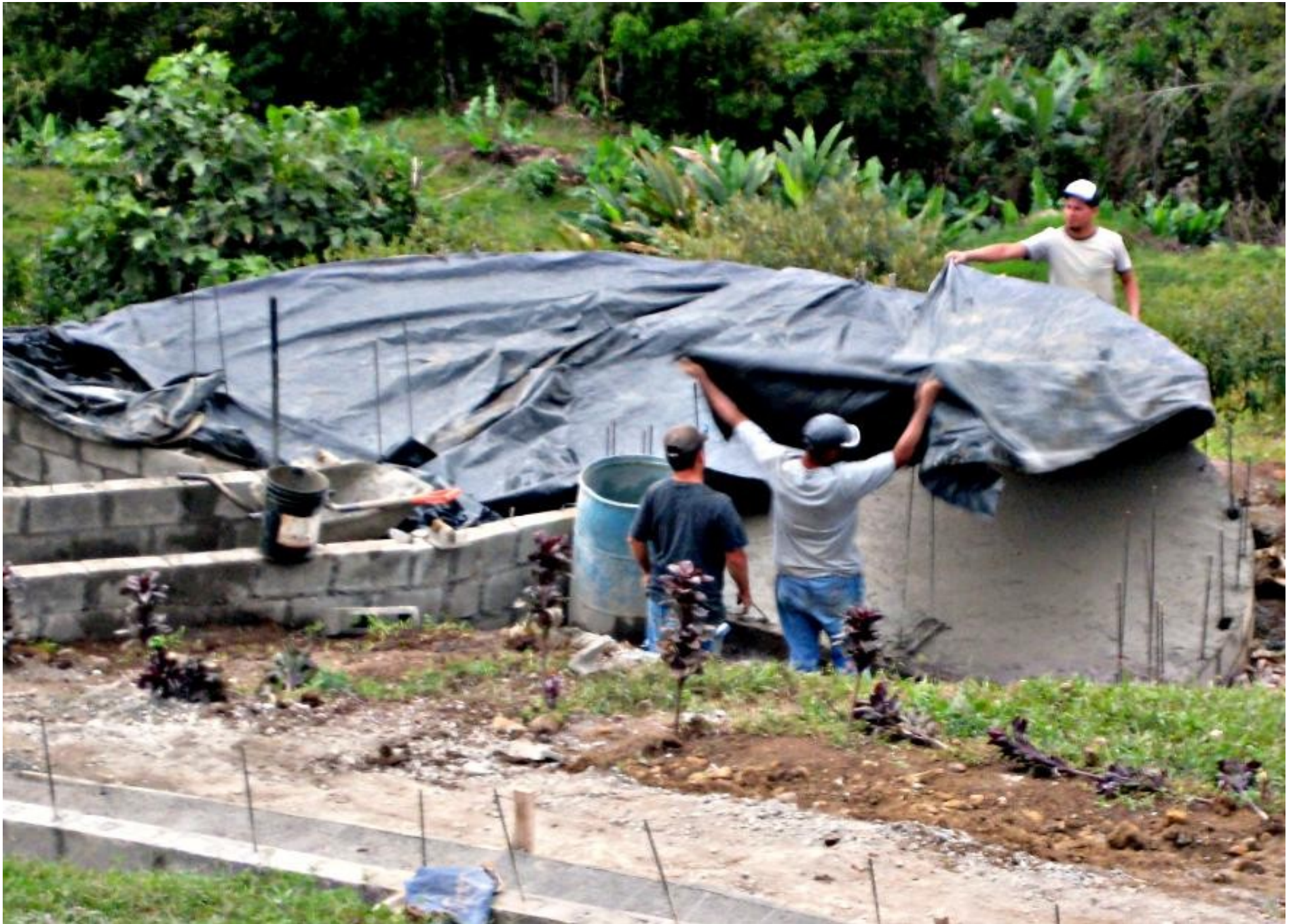
To protect the concrete from imminent rain.
