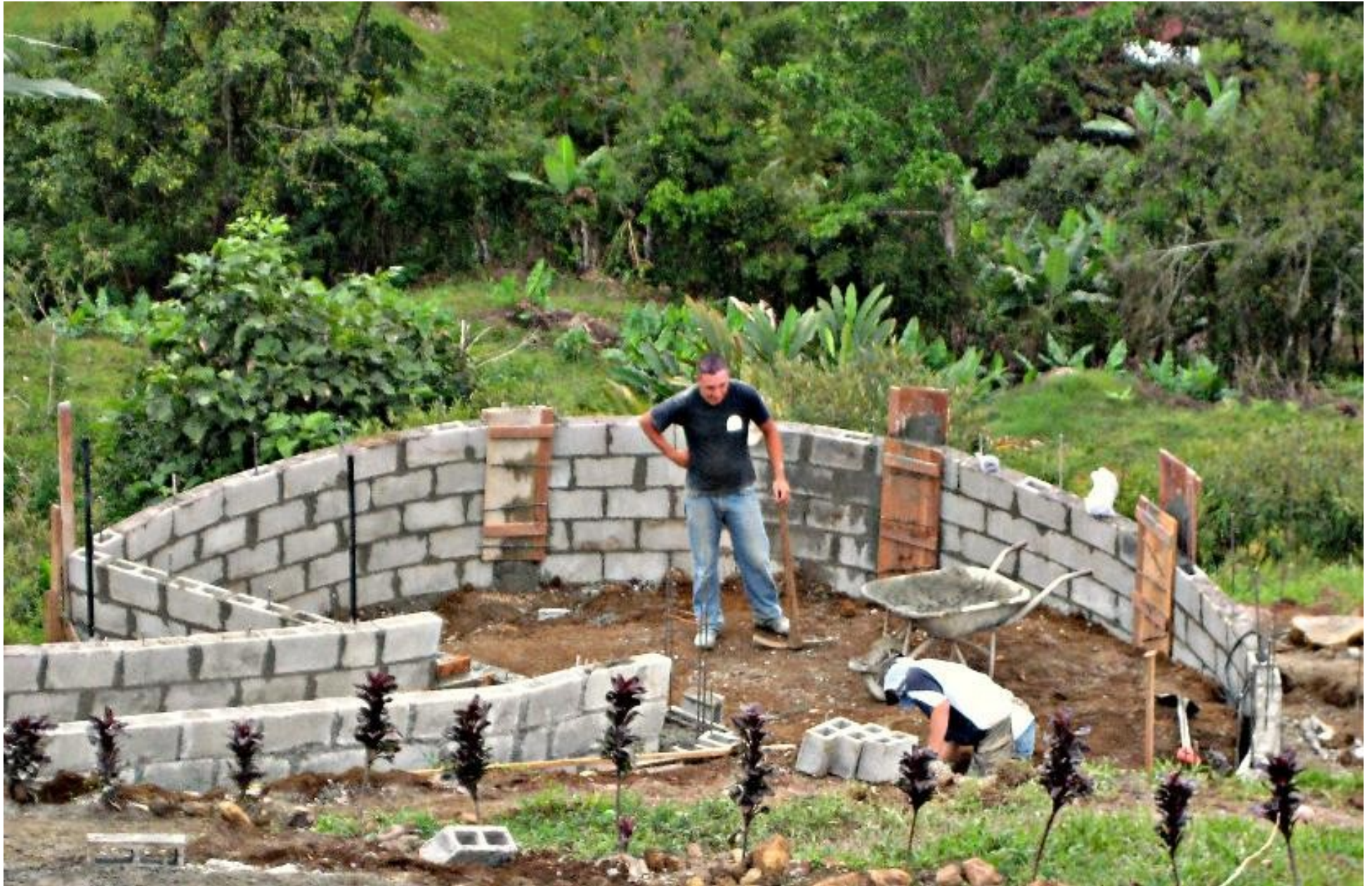
The rows block are interrupted to add strengthening rebar and concrete
